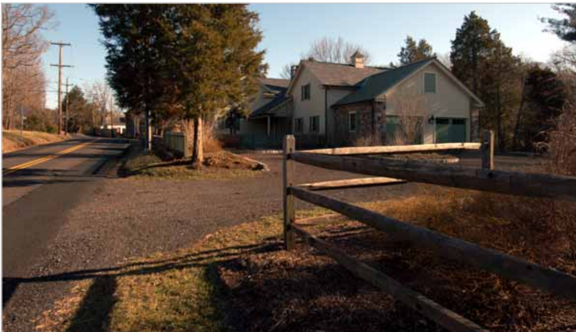
Figure 72. New driveway and parking area at the recently expanded dwelling on Aquetong Road, Carversville Historic District. Crushed stone paving is a compatible and environmentally friendly paving surface.
