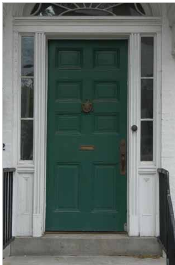
Figure 29. Federal style door with period hardware intact. The preservation of period hardware on historic doors is highly recommended.
