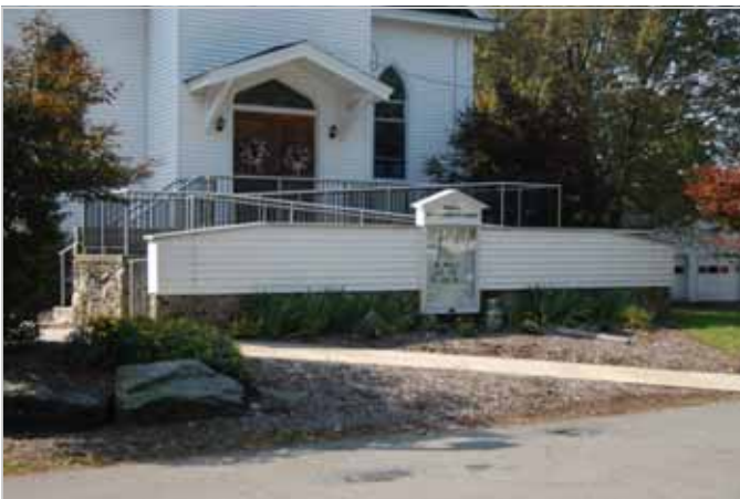
Figure 25a. Examples of unsuccessful ADA ramps. Left: The designer of the ramp in front of the historic wood frame church made an attempt to screen the long ramp, but because of the required length of the ramp, it should have been placed on the side of the building. Right: Pressure-treated wood railings and exposed structure are not recommended.
