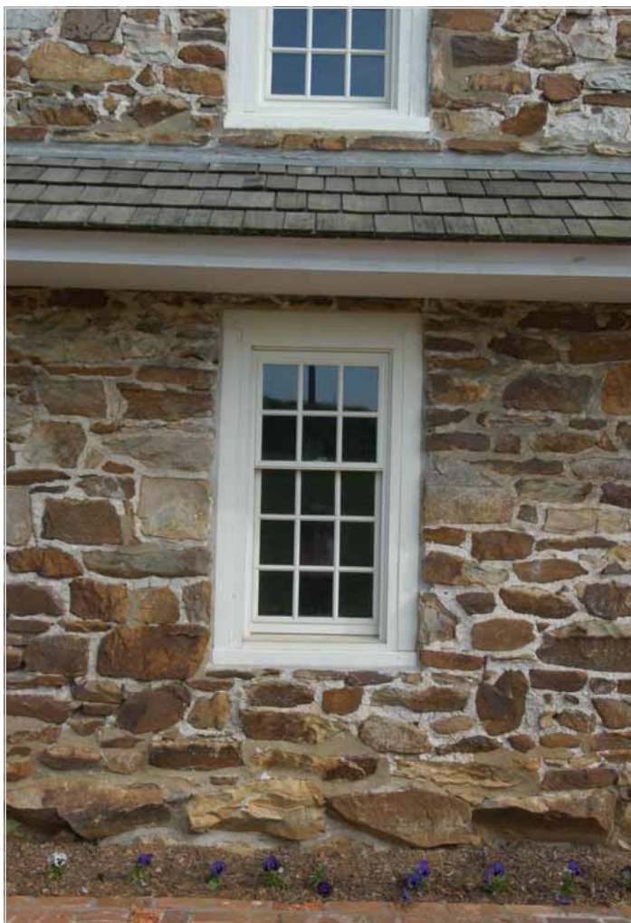
Figure 55. Standard size vinyl replacement windows fitted to window frames by means of wood filler strips destroy the original proportions of the windows and are not recommended.
