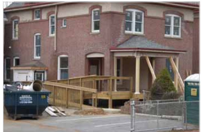
Figure 25a. Examples of unsuccessful ADA ramps. Left: The designer of the ramp in front of the historic wood frame church made an attempt to screen the long ramp, but because of the required length of the ramp, it should have been placed on the side of the building. Right: Pressure-treated wood railings and exposed structure are not recommended.
