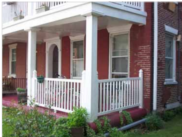
Figure 38. Left: Inappropriate porch alterations extended this historic porch outside of its roofline replaced the original railing with an interior railing system utilizing widely spaced, undersized, balusters. Right: Vinyl railing systems lack the detailing, scale, and finish of wood railing systems.
