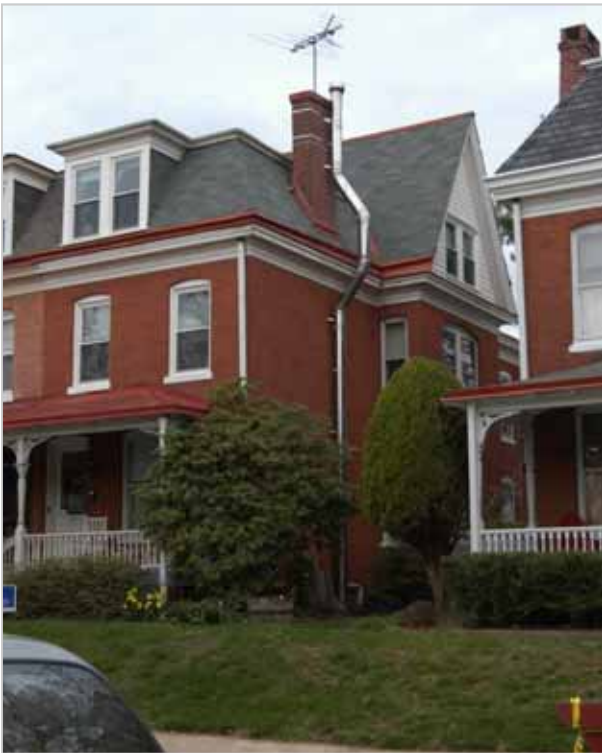
Figure 34. Left: Stainless steel flue run outside of chimney in a National Register-listed residence not located in a zoning historic district. Right: Restaurant kitchens are very intrusive to historic buildings. To reduce cost, exhaust fans for a commercial exhaust hood were run out the side of this Colonial Revival building instead of through the roof, and a massive electric service was brought to the building aerially.
