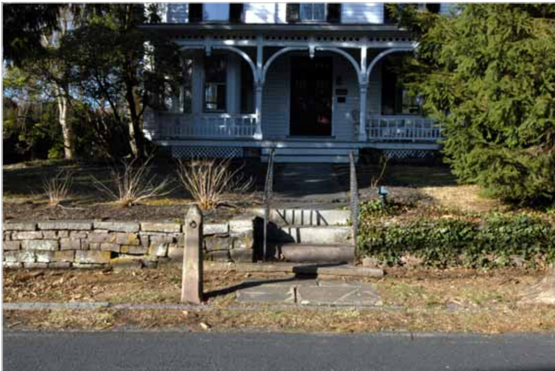
Figure 76. Paving along Aquetong Road, Carversville Historic District. Note the surviving bluestone curbing, dry-laid retaining wall, flagstone sidewalk and walk to the porch, and hitching post.
