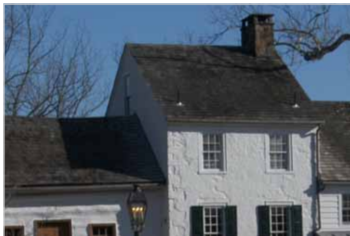
Figure 48. Kirk Homestead, Carversville Historic District. Because of the prominence of the roofs of colonial vernacular houses, the preservation of historic wood shingle roofing is especially important.
