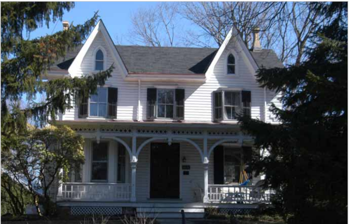
Figure 10. Gothic Revival house along Aquetong Road, Carversville Historic District. The cross gables, steeply-pitched roof, chimney pots, and ornamental porch framing are characteristics of the Gothic Revival style.
