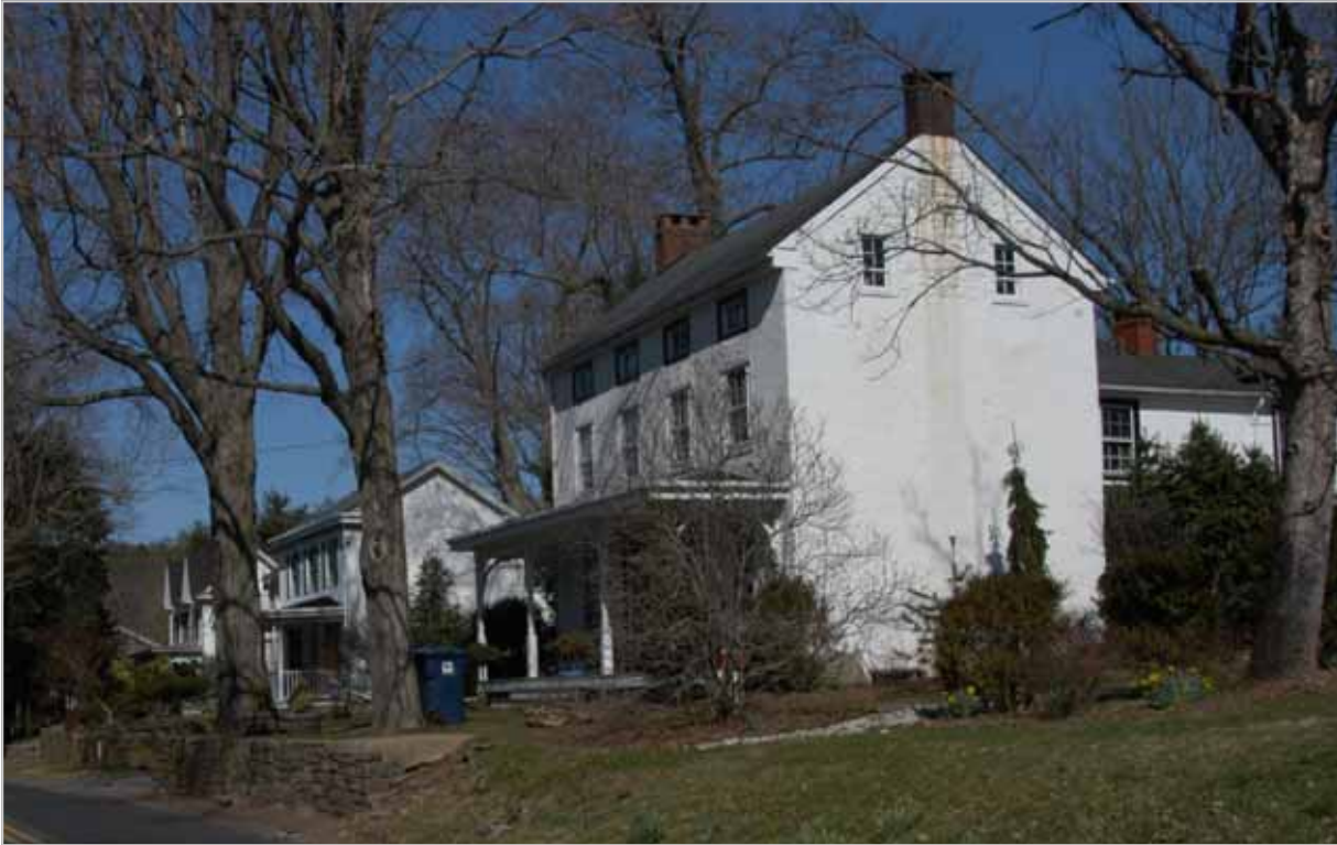
Figure 6b. Aquetong Road, Carversville Historic District. Dwellings in Carversville are generally simple masses, two and one-half stories in height, with gable roofs.
