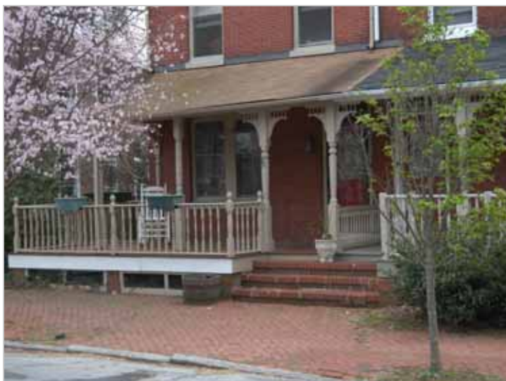
Figure 38. Left: Inappropriate porch alterations extended this historic porch outside of its roofline replaced the original railing with an interior railing system utilizing widely spaced, undersized, balusters. Right: Vinyl railing systems lack the detailing, scale, and finish of wood railing systems.
