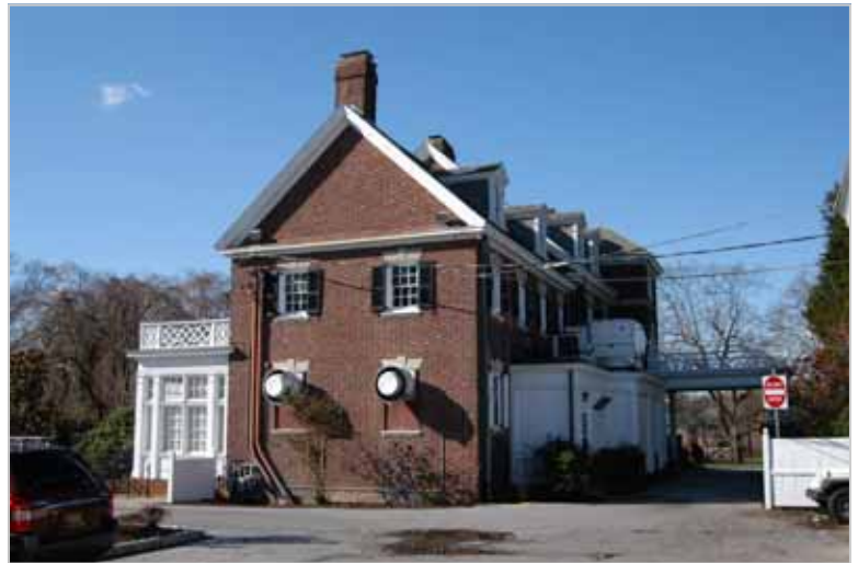
Figure 34. Left: Stainless steel flue run outside of chimney in a National Register-listed residence not located in a zoning historic district. Right: Restaurant kitchens are very intrusive to historic buildings. To reduce cost, exhaust fans for a commercial exhaust hood were run out the side of this Colonial Revival building instead of through the roof, and a massive electric service was brought to the building aerially.
