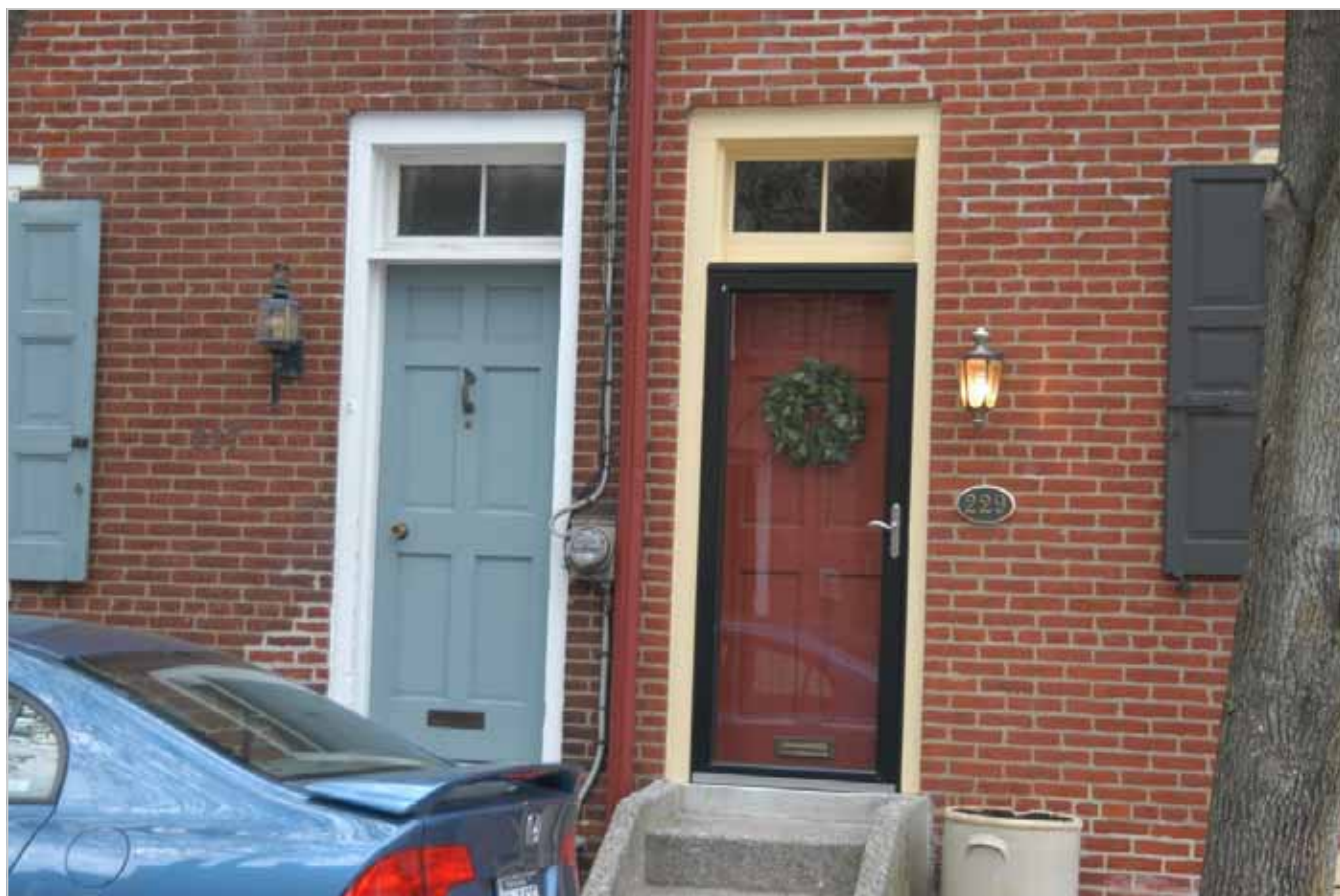
Figure 30. On the left is a historic wood door without the protection of a storm door. The aluminum storm door at the right entrance allows a view of the historic wood door through its large, simple glass panel with negligible visual impact.
