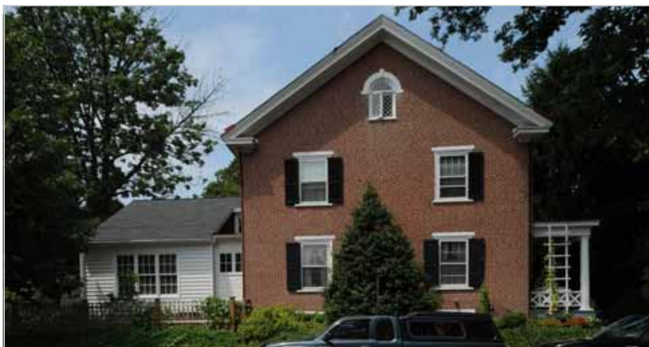
Figure 64. The ridge line and cornice line of an addition should be lower than the ridge line and cornice line of the original structure, and the volume of the addition should be less than that of the primary structure.
