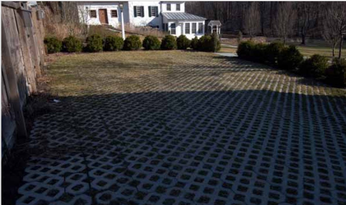
Figure 71. Parking area at the Kirk Homestead, Aquetong Road, Carversville Historic District. Grassblock pavers are successfully employed where the amount of automobile parking is not heavy.
