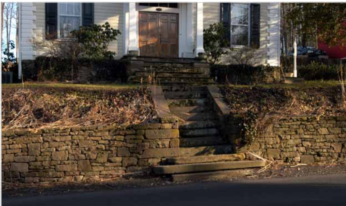
Figure 75. One of the more formal retaining walls and entrance steps in the Carversville Historic District is found at the Samuel and Hannah Firman House on Carversville Road. Note the stone walls, stone slab steps, and stone walk.
