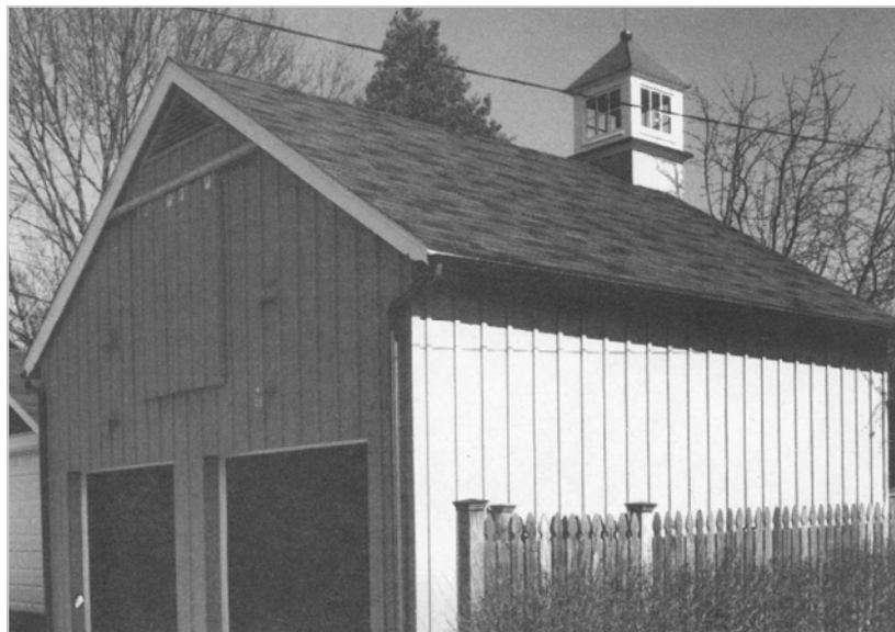
Figure 66. Example of a new garage that is compatible with its historic setting through the use of traditional board-and-batten siding, gabled roof form, storage loft, and placement on the lot.
