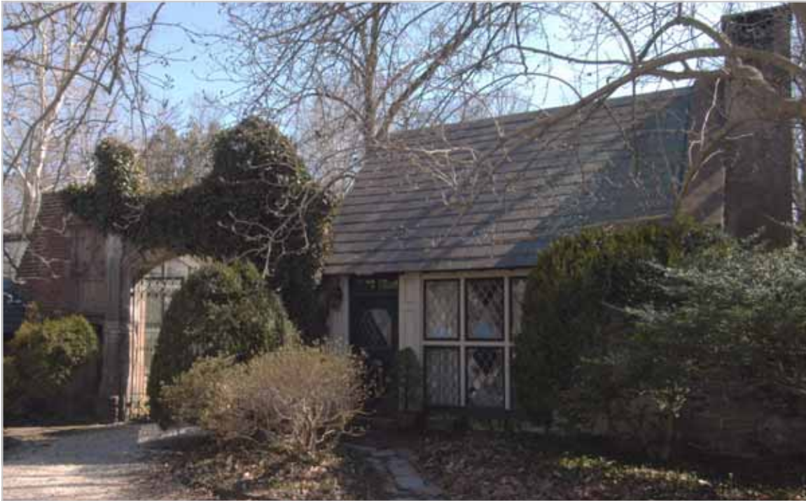
Figure 13a. Whimsical Tudor Revival style outbuilding and gateway attached to the Morgan Colt House, Phillips Mill Historic District. Phillips Mill achieves its uniqueness and significance from its eclectic blend of Tudor Revival influences, gothic motifs, and arts-and-crafts motifs, applied to otherwise substantial, but typical, colonial and nineteenth-century buildings.
