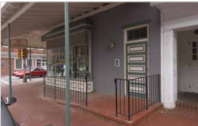
Figure 25b. Examples of successful ramps. Left: The shop entrance requires only a short ramp and the use of brick paving masks the presence of the ramp. Right: Porches provide a natural screen for a new ramp.
