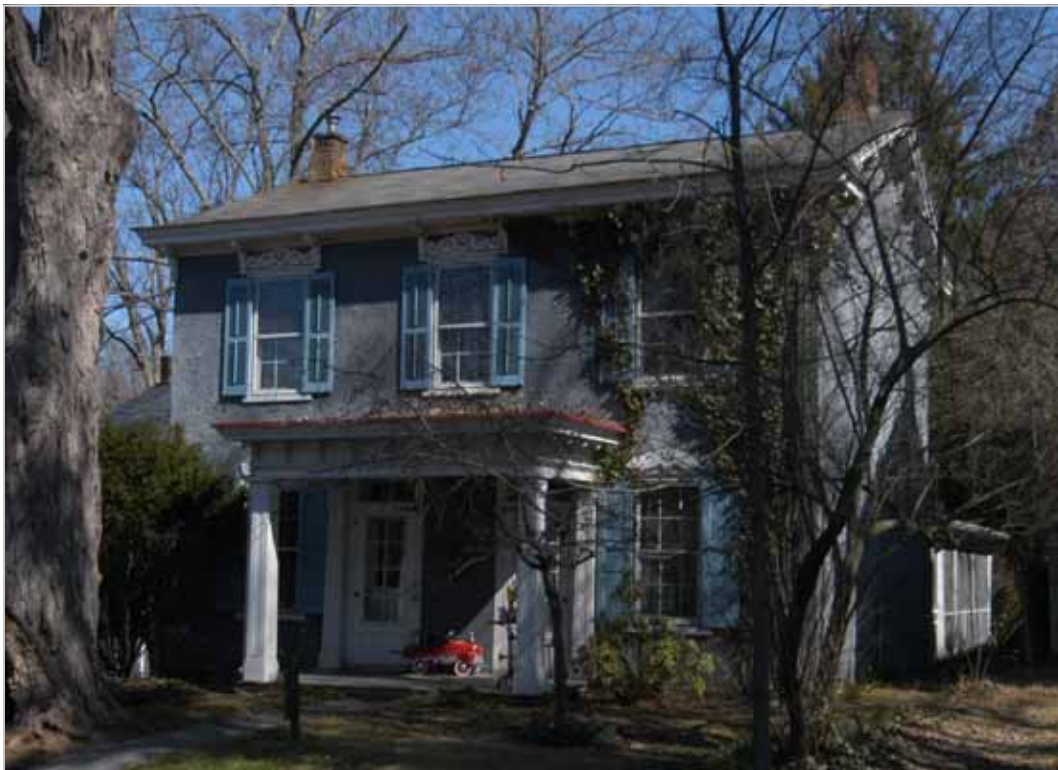
Figure 11. Italianate style house on Aquetong Road, Carversville Historic District. The bracketed cornice, wide overhangs, and porch are hallmarks of the Italianate style.
