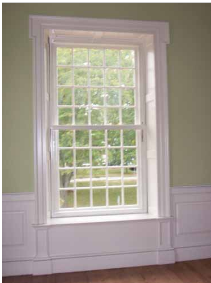
Figure 58. Interior storm window glazed with clear glass.
