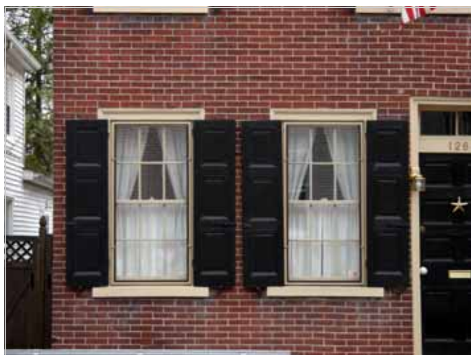
Figure 57. Three-track storm window with stock color finish. For one-over-one double-hung sash windows, three-track storms are a recommended treatment.
