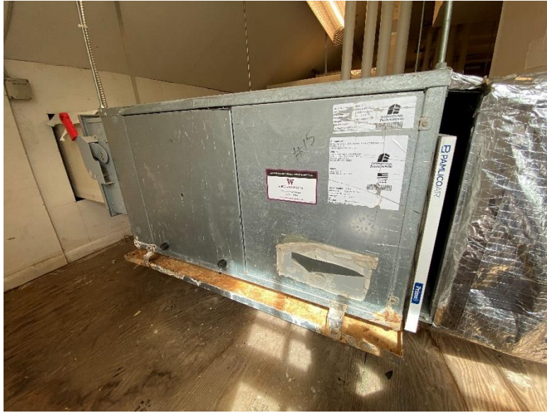
Fan Coil Unit FC-15
