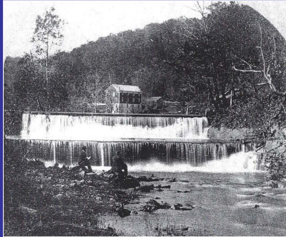
Wall Mill Dam
