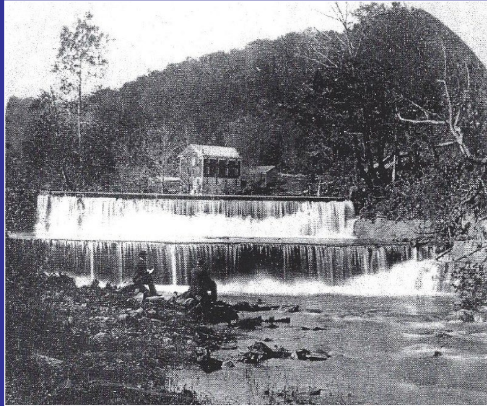
Wall Mill Dam
