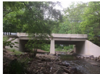
STRUCTURAL AND FORENSIC
