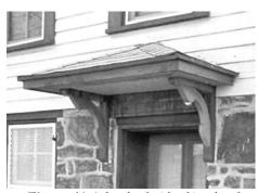
Figure 64 A door hood with a hipped roof
