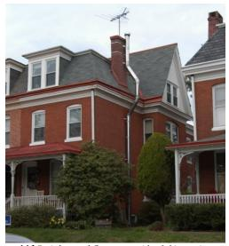
Figure 146 Stainless steel flue run outside of chimney in a National Register-listed residence not located in a zoning historic district.
