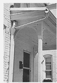
Figure 201 A gutter and downspout
