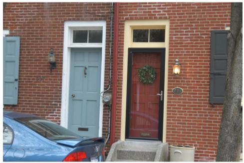
Figure 142 On the left is a historic wood door without the protection of a storm door. The aluminum storm door at the right entrance allows a view of the historic wood door through its large, simple glass panel with negligible visual impact.
