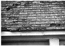
Figure 73 Deteriorating slate roof
