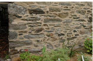
**Figure 145** Overly-hard Portland cement mortar restrains the expansion of permeable stone masonry and results in the delamination (loss) of the face of the stone.
