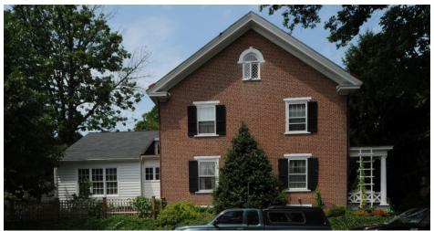
**Figure 180** The ridge line and cornice line of an addition should be lower than the ridge line and cornice line of the original structure, and the volume of the addition should be less than that of the primary structure.
