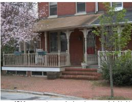
Figure 151 Inappropriate porch alterations extended this historic porch outside of its roofline replaced the original railing with an interior railing system utilizing widely spaced, undersized, balusters.
