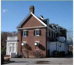
Figure 147 Restaurant kitchens are very intrusive to historic buildings. To reduce cost, exhaust fans for a commercial exhaust hood were run out the side of this Colonial Revival building instead of through the roof, and a massive electric service was brought to the building aerially.
