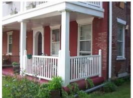
Figure 152 V inyl railing systems lack the detailing, scale, and finish of wood railing systems.
