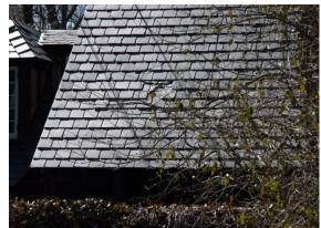
Figure 162 Slate roof in Phillips Mill residence. Although a few slates in the center have been broken by mechanical damage (probably a tree limb), replacement of the broken slates is readily accomplished without disturbing surrounding slates.
