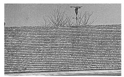
Figure 74 Wood shingle roof
