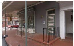
Figure 136 Successful ramp: The shop entrance requires a short ramp and the use of brick paving masks the presence of the ramp
