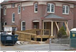
Figure 135 Unsuccessful ramp. The pressure-treated wood railings and exposed structure are not recommended
