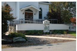
**Figure 134** Unsuccessful ramp in front of historic wood frame church. The designer attempted to screen the long ramp, but it should have been placed on the side of the building due to its length
