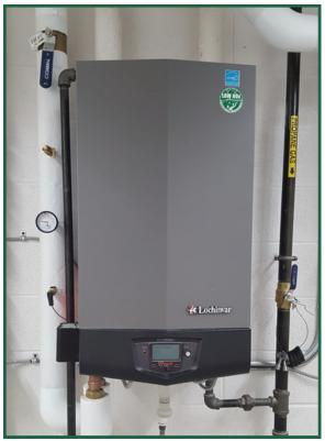
SMALL BUT MIGHTY, this unassuming gray box, hanging on a wall inside the new Public Works building, will heat all 14,000-square-feet of the structure. It warms water that is continuously recycled in a closed-loop system, circulating it through tubing embedded in the facility
