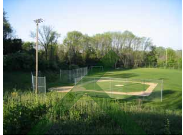
Existing Field Lighting
