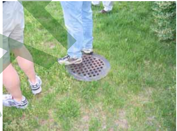
Existing Stormwater Inlet, Lower Park Area
