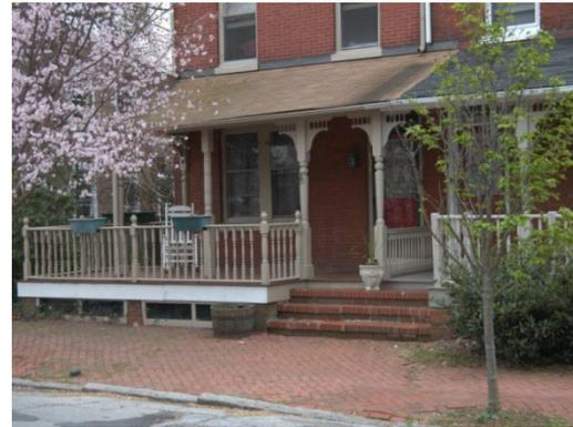
**Figure 151** Inappropriate porch alterations extended this historic porch outside of its roofline replaced the original railing with an interior railing system utilizing widely spaced, undersized, balusters.
