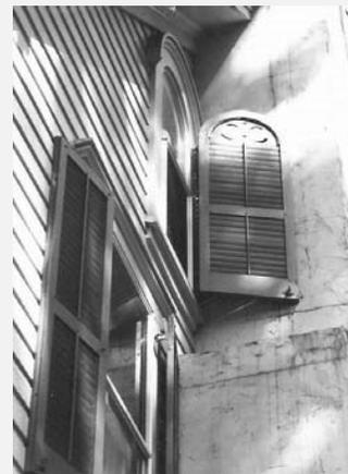
*Figure 20 Detail of attic shutter from Shaw house*
