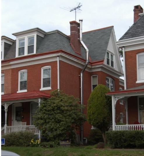
**Figure 146** Stainless steel flue run outside of chimney in a National Register-listed residence not located in a zoning historic district.
