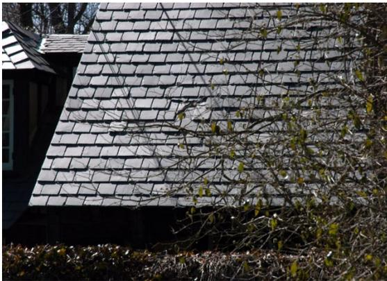
**Figure 162** Slate roof in Phillips Mill residence. Although a few slates in the center have been broken by mechanical damage (probably a tree limb), replacement of the broken slates is readily accomplished without disturbing surrounding slates.
