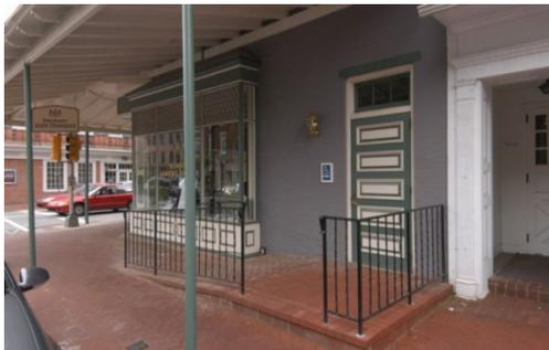
**Figure 136** *Successful ramp: The shop entrance requires a ramp and the use of brick paving masks the presence of the ramp*
