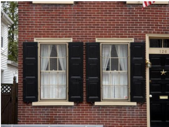
**Figure 173** Three-track storm window with stock color finish. For one-over-one double-hung sash windows, three-track storms are a recommended treatment.
