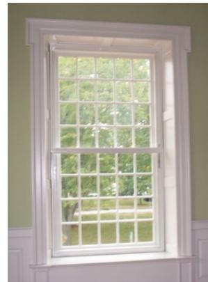
**Figure 174** Interior storm window glazed with clear glass.
