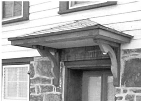
*Figure 64 A door hood with a hipped roof*
