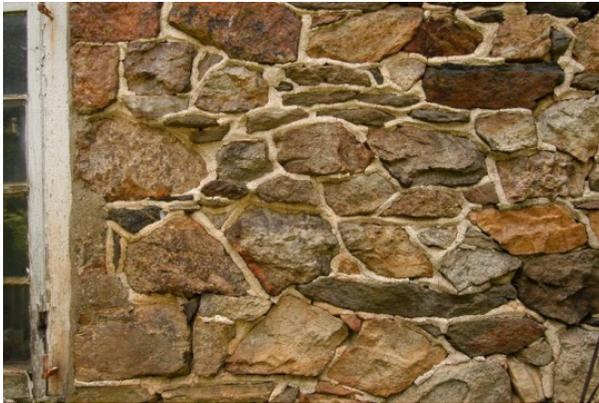
**Figure 144** Detail of eighteenth century pointing. The most common joint profile type for rubble stone masonry was the raised ridge joint.
