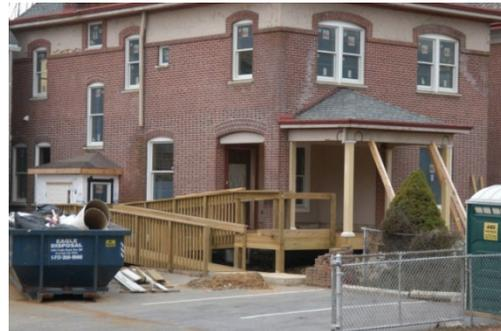
**Figure 135** *Unsuccessful ramp. The pressure-treated wood railings and exposed structure are not recommended*
