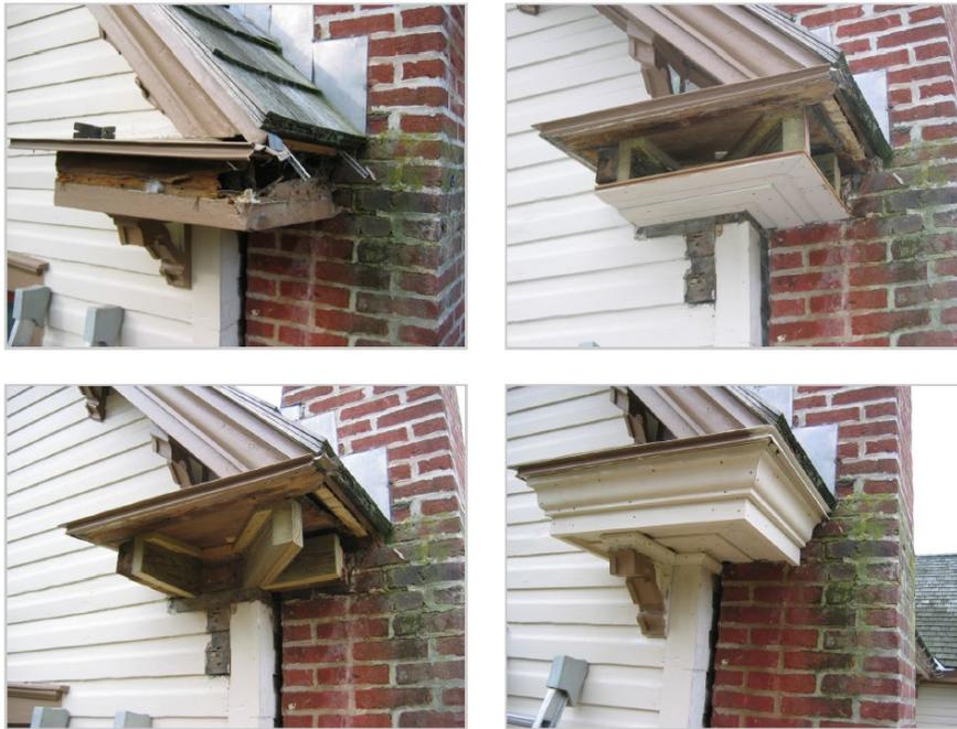
*Figure 133* Sequence of restoration of a severely deteriorated cornice return. The crown molding was custom-cut for the project, a procedure that requires scheduling but does not add significantly to the repair cost.
