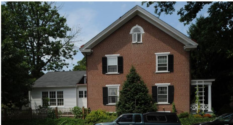
**Figure 180** The ridge line and cornice line of an addition should be lower than the ridge line and cornice line of the original structure, and the volume of the addition should be less than that of the primary structure.
