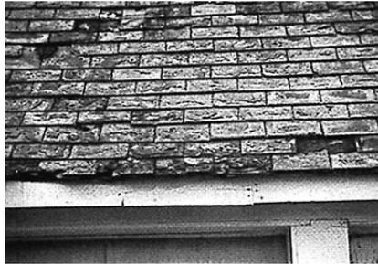
*Figure 73 Deteriorating slate roof*
