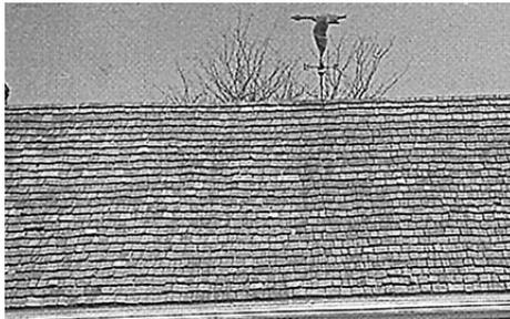
*Figure 74 Wood shingle roof*
