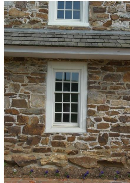
**Figure 170** Standard size vinyl replacement windows fitted to window frames by means of wood filler strips destroy the original proportions of the windows and are not recommended.
