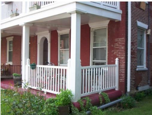
**Figure 152** Vinyl railing systems lack the detailing, scale, and finish of wood railing systems.
