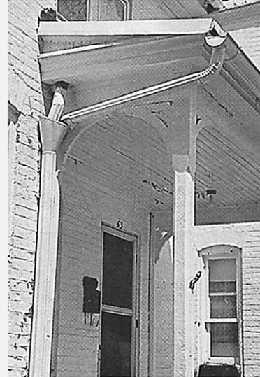
*Figure 201 A gutter and downspout*
